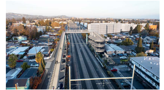
Aerial view of bridge facing west
