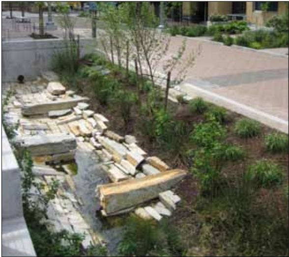
*Creative on-site retention facilities to detain, treat and reuse stormwater for irrigation are required for new development*
