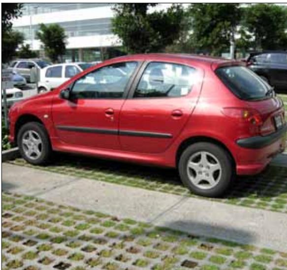
*New development can incorporate permeable paving in surface parking areas that allow stormwater infiltration*
