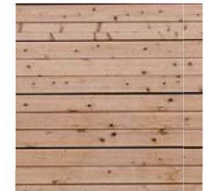
SIDING 1X6 ROUGH-SAWN CEDAR, OR REDWOOD HORIZONTAL PLANK, W/ REVEAL EVERY THIRD BOARD
