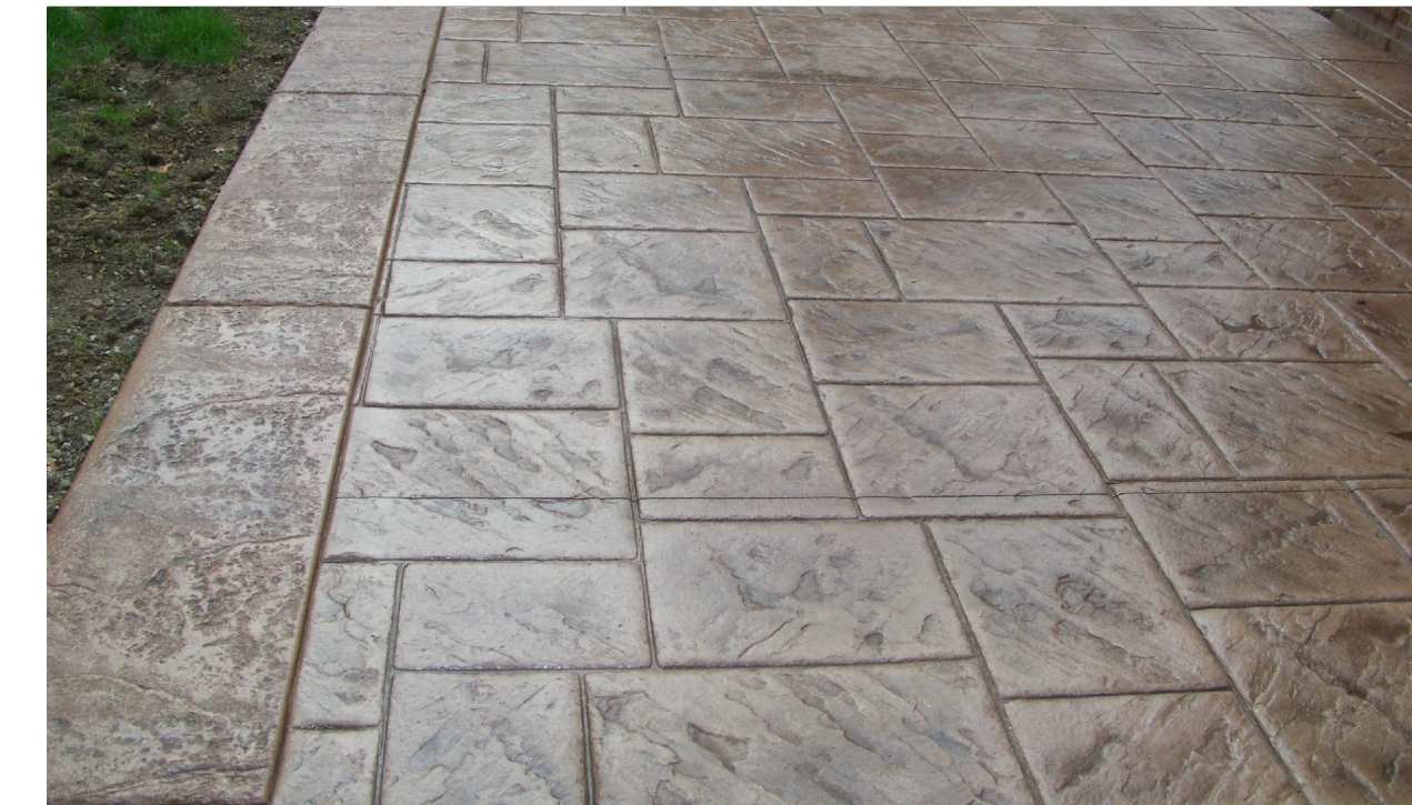
STAMPED CONCRETE AT DRIVEWAY ENTRANCES
