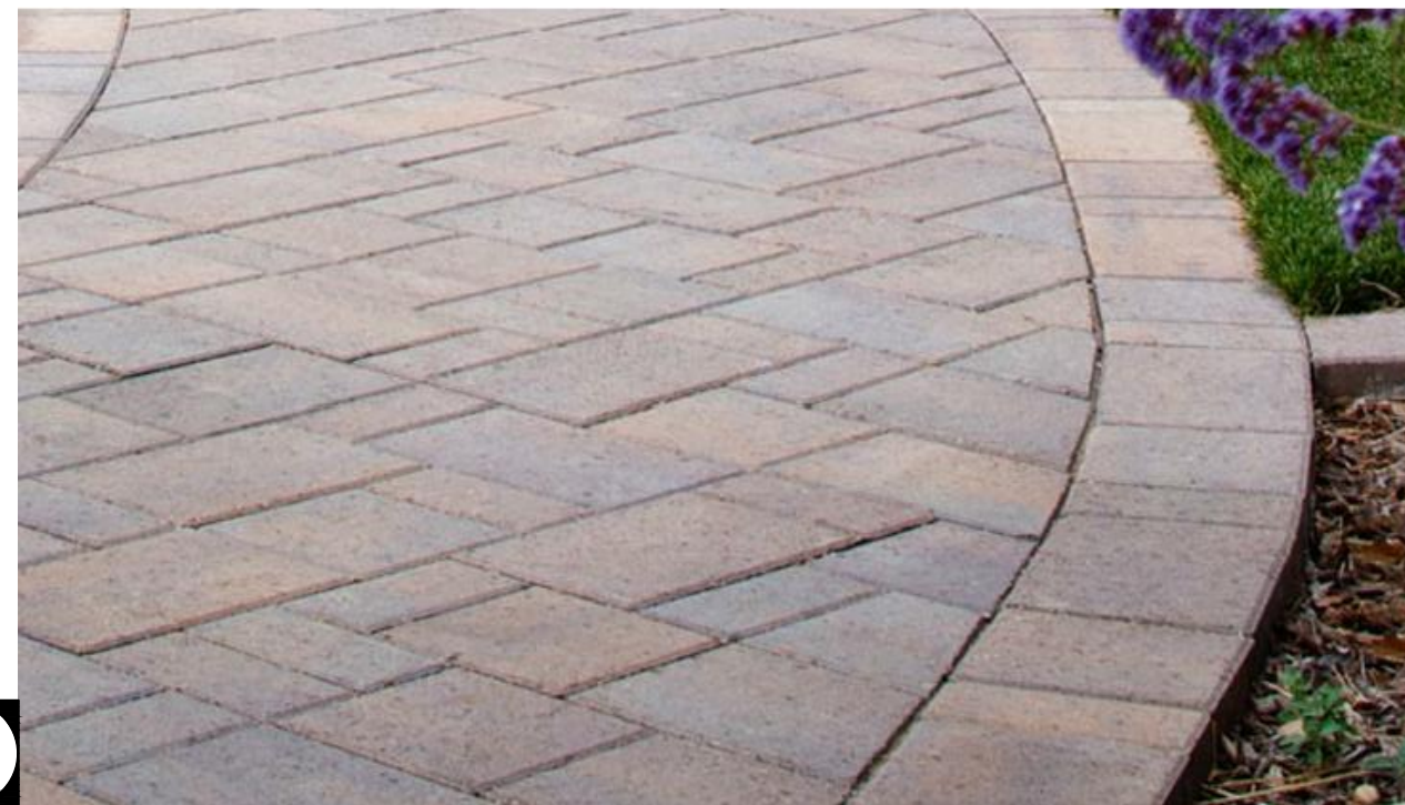
PERMEABLE PAVERS AT DRIVEWAYS (ASHLAR PATTERN)
