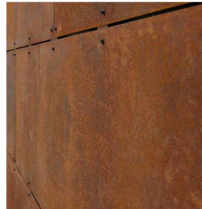
CORTEN STEEL PLATE AT ENTRY GATE AND GABION BENCH
