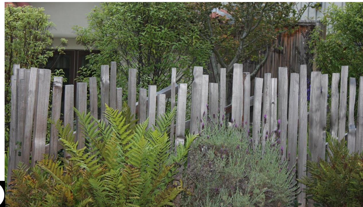
GRAPE STAKE FENCE AT BLUFF TRAIL (18' HEIGHT, TYP. W/ IRREGULAR PICKETS, FLAT TOP)
